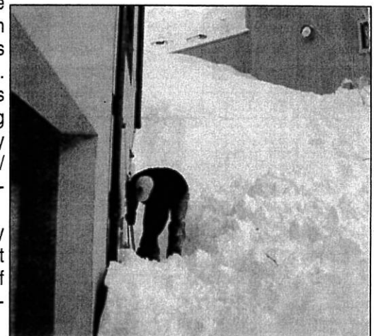
Concerns were raised for external gas lines exposed to burial and damage by avalanche debris.
